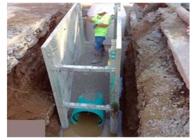
Under Main St: Placing the new sewer pipe.
