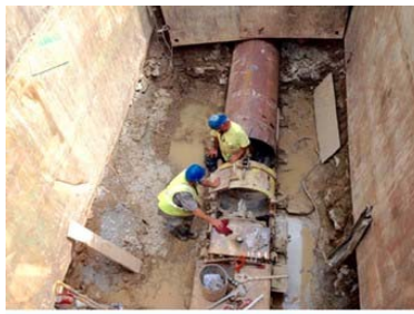
Inside the Pit at Short St: Tunneling Under Midland Ave
